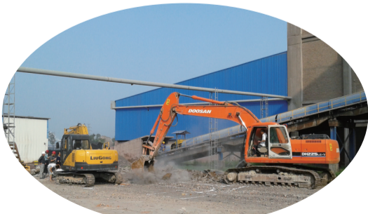
挖掘机开挖基槽
